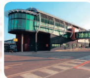
KING SHAKA INTERNATIONAL AIRPORT
