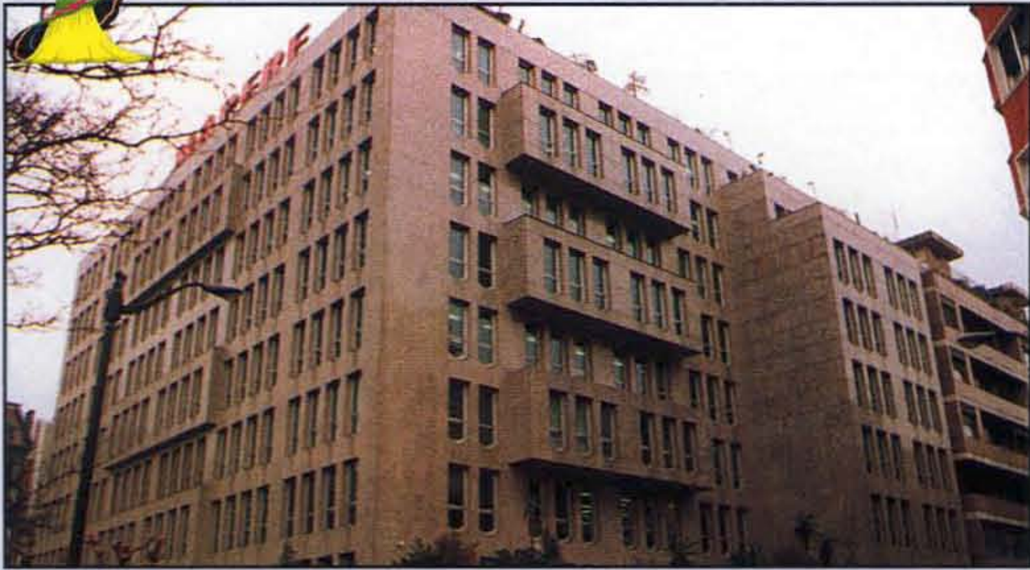
MSC's offices in Bilbao are situated on the 4th floor of this imposing building
