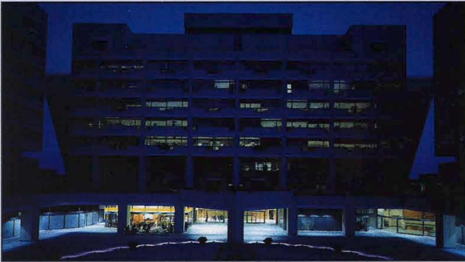
MSC's offices are situated on the 8th floor of the World Trade Centre adjacent to the Barcelona Passenger Ship Terminal
