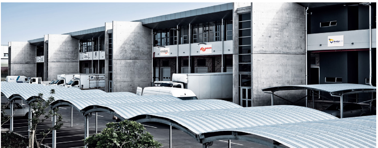
Dube TradeHouse is central to the TradeZone freight operations and offers integrated warehousing and office space.
